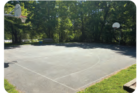
The Glen Mar Neighborhood Park basketball court before (above) and after (top).
